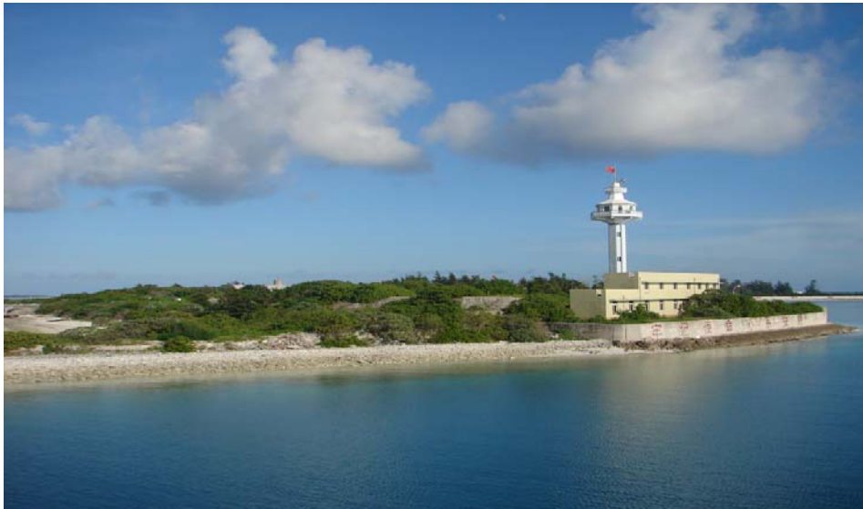
Duncan, Communication Tower
